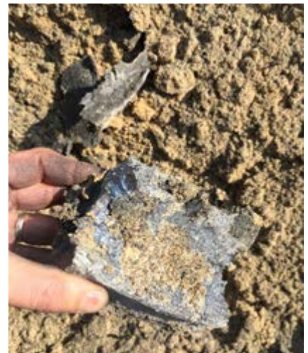
Cutting Steel: NX5600 charge used, 65mm severed
